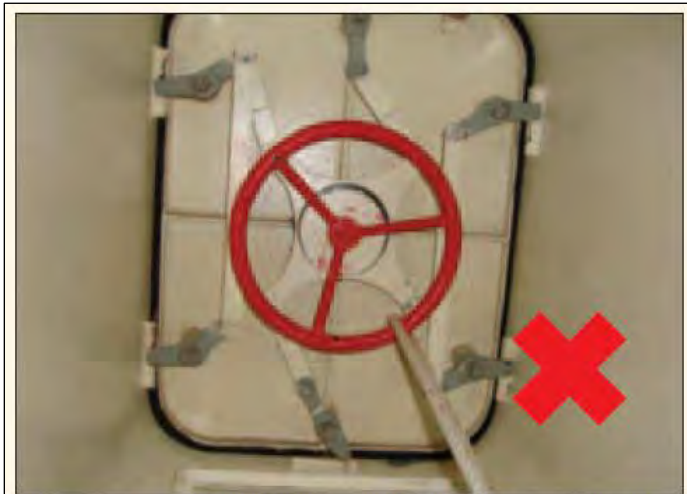
▲ Figure 1: Hatch tied down with rope may be unopenable from outside for entry during fire-fighting operations
